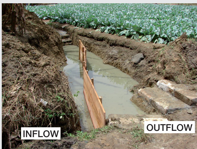
Figure 4: Interconnected pond with hardwood baffle.
