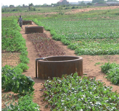
Figure 2: Interconnected tank system in Lomé, Togo (the water source here is shallow groundwater).
