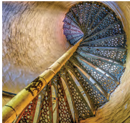
The Beaver Island Lighthouse School property is owned by Charlevoix County and Networks Northwest. The Lighthouse on this property is a cultural resource, as described in Chapter 2.
