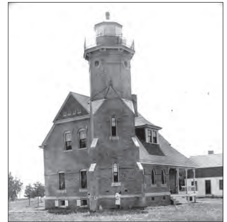
One of the privately-owned islands in the Archipelago, Ojibwa Island is renowned for its historic lighthouse built in 1892. A work crew from Beaver Island performed significant preservation work on the lighthouse in 2016. Photo Credit: US Coast Guard Archives
