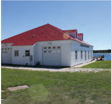
The CMU Boathouse is an easily recognizable building located on Paradise Bay.
